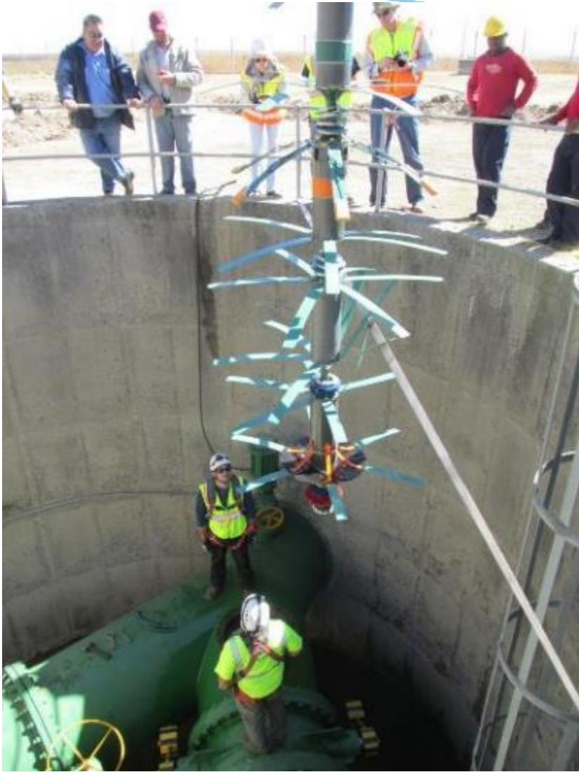
PipeDiver (Operating Pipeline)
