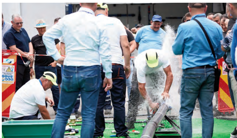
Fig. 9 - Concurs „Instalare bransament sub presiune” / “Installing a connection under pressure” Contest
